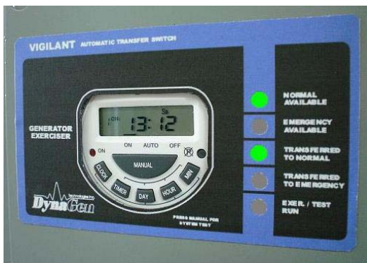
Correct LED alignment
