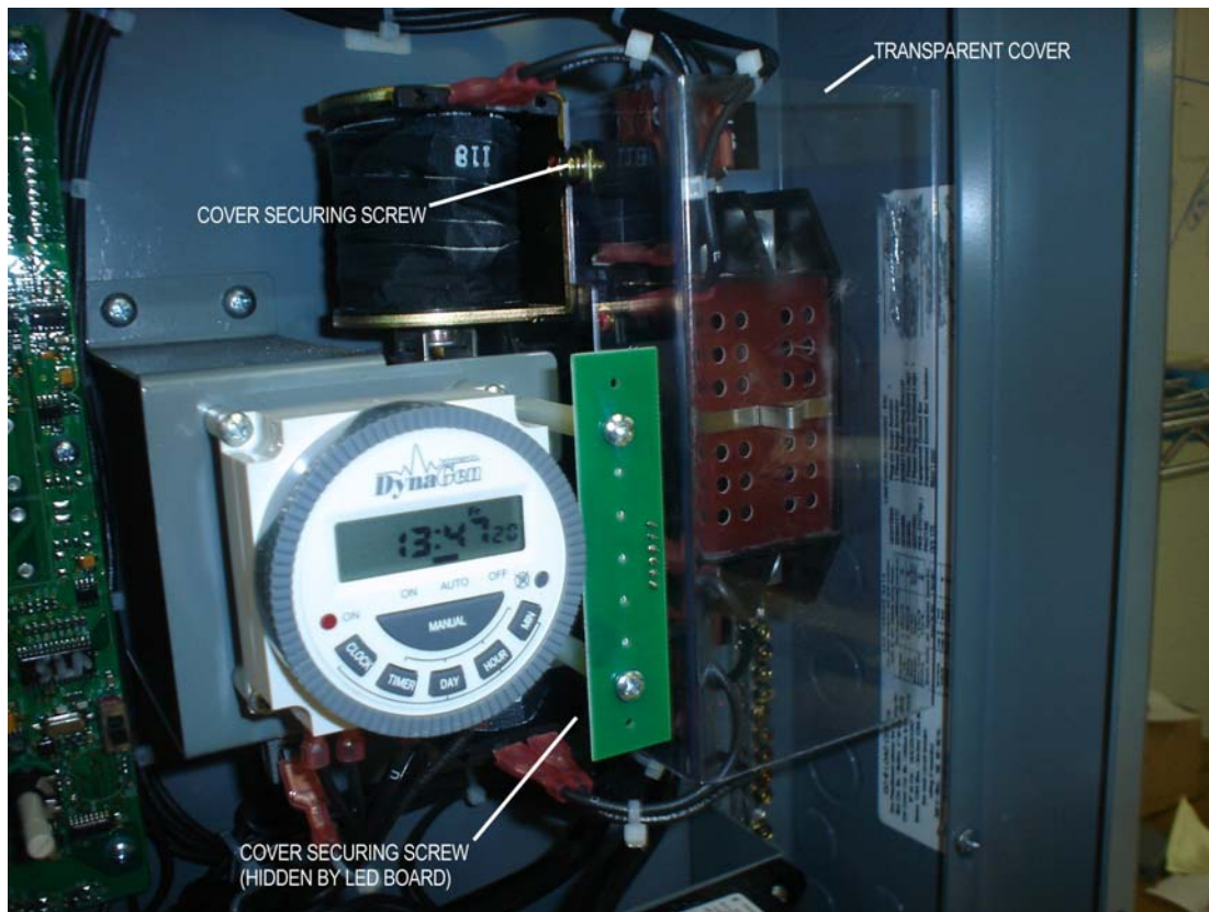
Figure 4. TRANSPARENT COVER SECURING SCREWS
