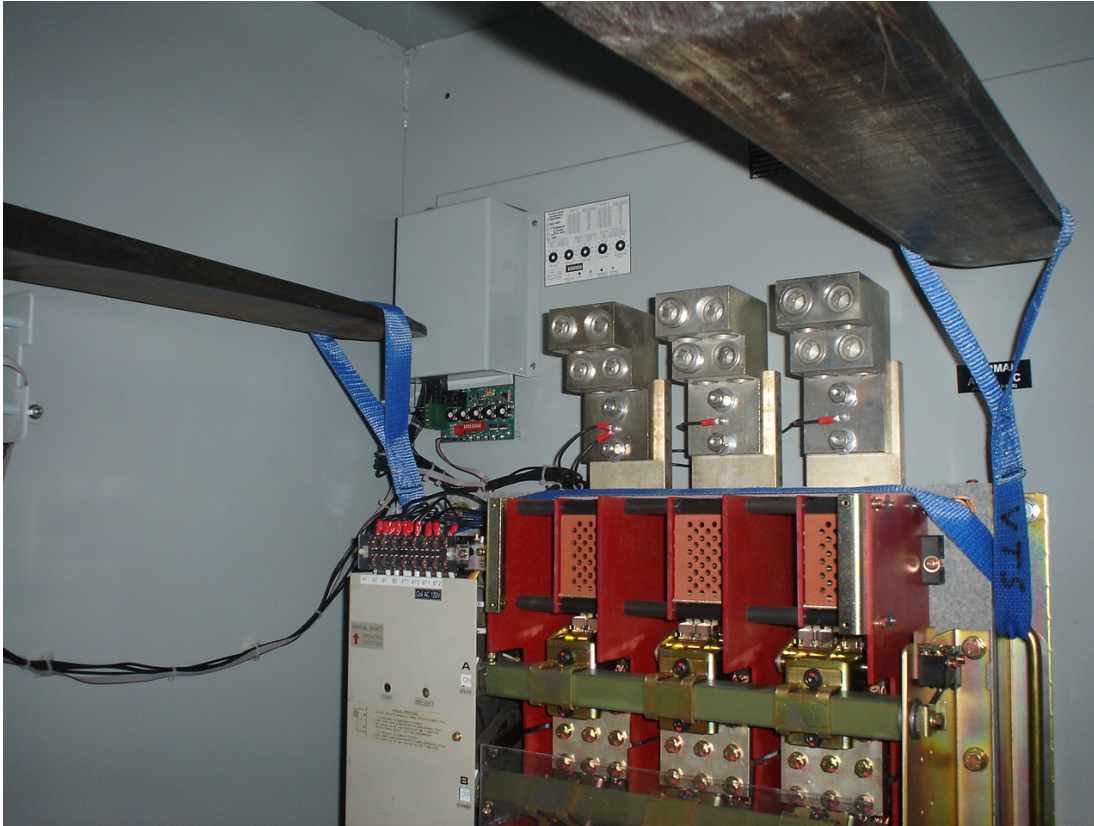
Figure 5. SWITCH REMOVAL
