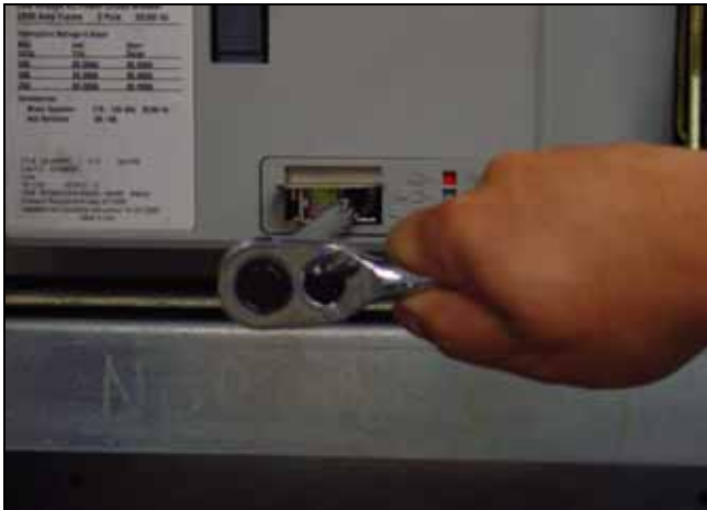
Figure 12. Levering and Position Indication.
