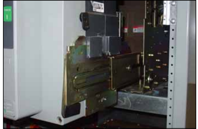
Figure 7. Switching Device in the REMOVE Position.
