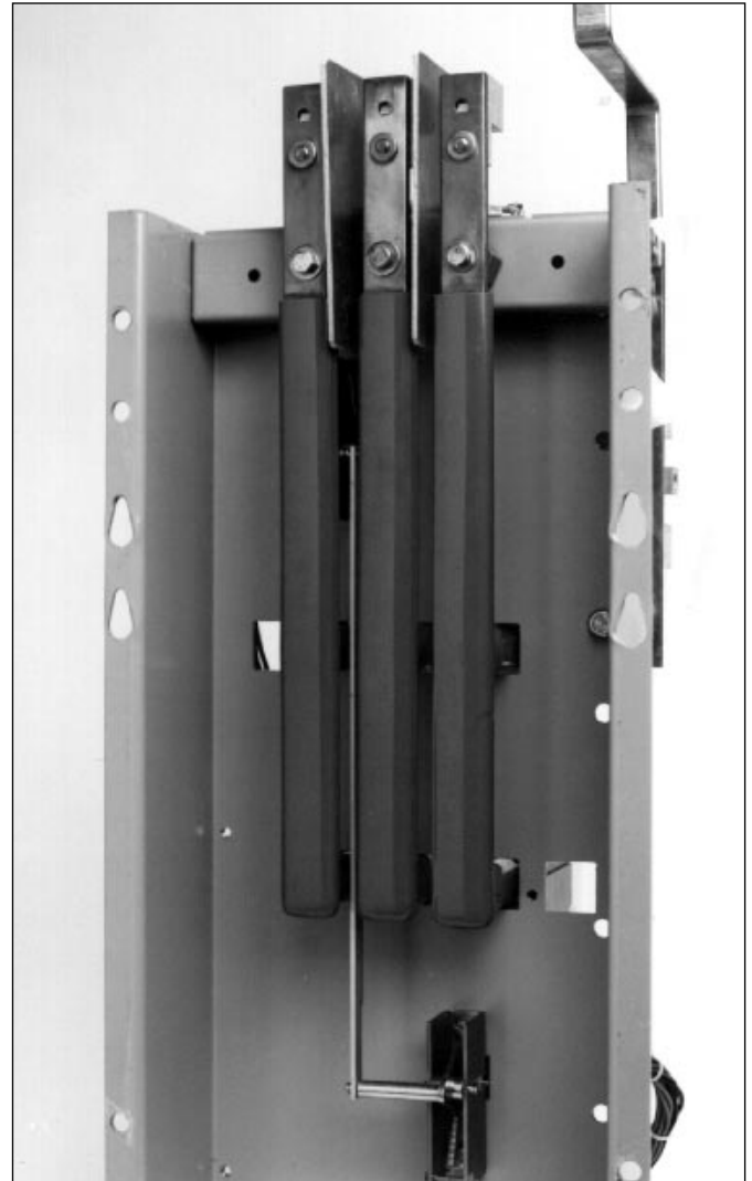
Figure 4-4 Mounted Load Lug Assembly (225-1000A Models)
